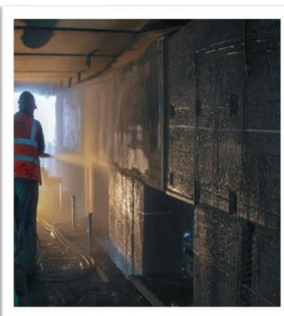
**The outcome:** The works were successfully completed with the ICCP System being commissioned and working well to provide ongoing protection to the support structures from future corrosion. The deteriorated concrete was repaired, and the sprayed concrete overlay successfully encapsulated the ICCP system and provided an improved aesthetic finish.
